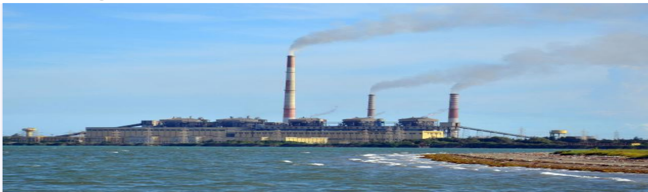
The Hindu A view of the Thermal Power Station in Tuticorin. Photo: N. Rajesh
